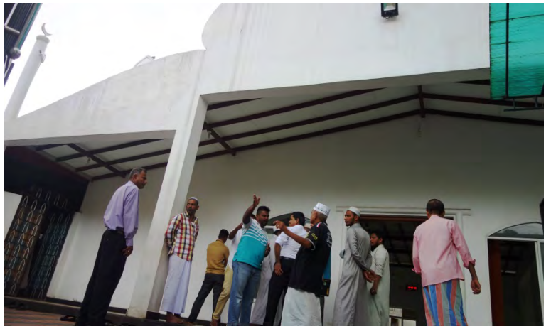
Above: the rebuilt mosque after it was destroyed by BBS supporters
